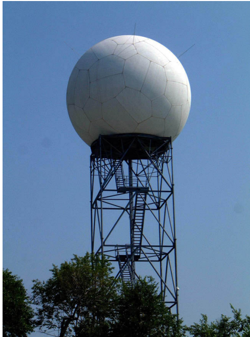
Figure 3. Typical NEXRAD Installation
