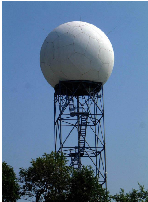
Figure 3. Typical NEXRAD Installation
