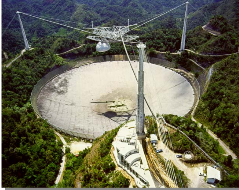
NSF's Arecibo Observatory, south of Arecibo, Puerto Rico. At 305 meters in diameter, Arecibo is by far the largest single-dish radio telescope in the world. It is used for radio astronomy, atmospheric/ionospheric research, and as a giant radar transmitter for mapping the structure of the Moon and planets. The telescope operates at various frequencies between 50 MHz and 10 GHz. Arecibo is operated by the National Astronomy and Ionosphere Center/Cornell University. (Photo courtesy NSF/NAIC/Cornell University).
