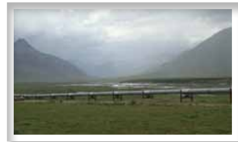
Truck on pipeline access road, north of Atigun Pass
