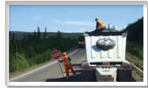
Road construction north of Livengood
