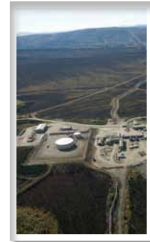
Pump Station 5 Photo by Steve Hillebrand/USFWS
