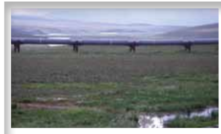
Trans-Alaska Pipeline between pump stations 2 and 3
